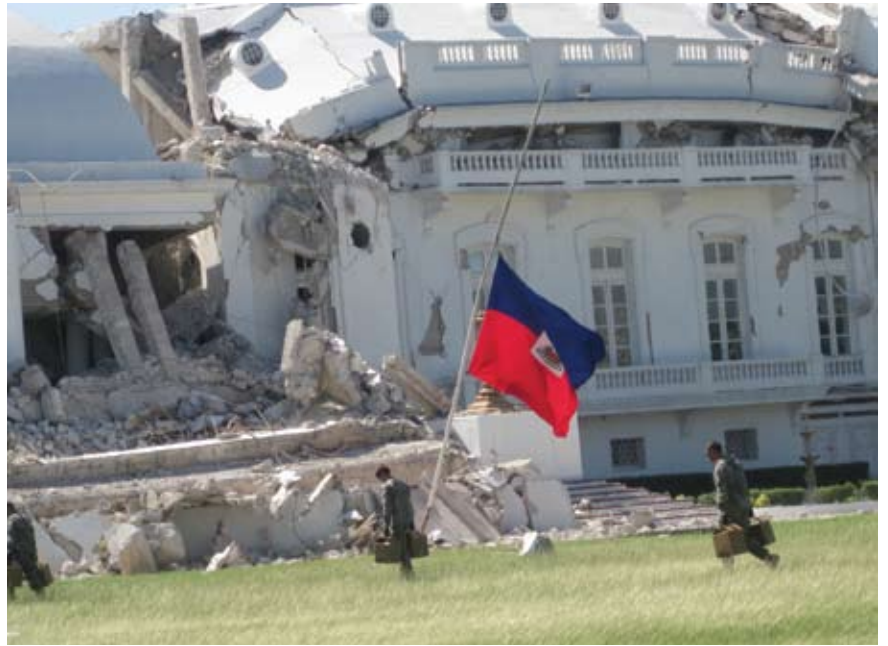
Significant damage to The Palace
