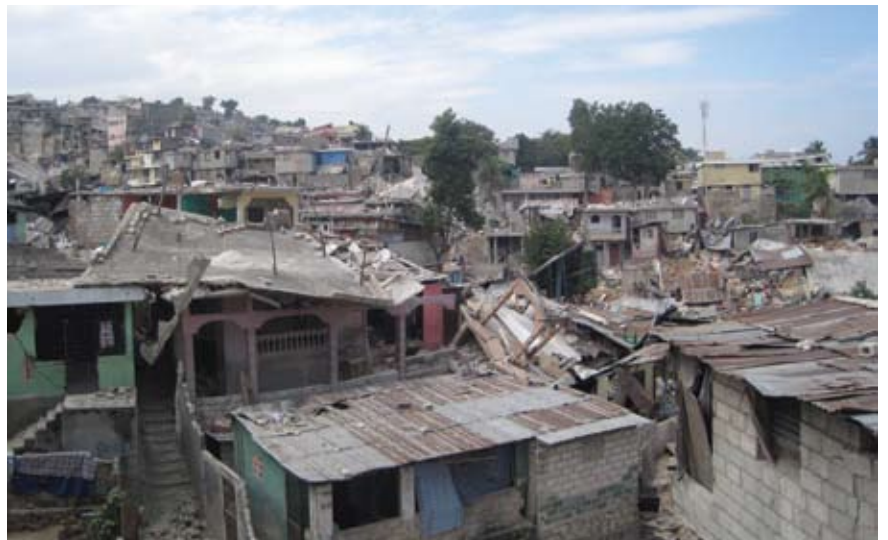
The earthquake left significant damage to many area neighborhoods.
